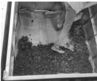
Plate 4. Installation of the Outer and Inner Tanks
